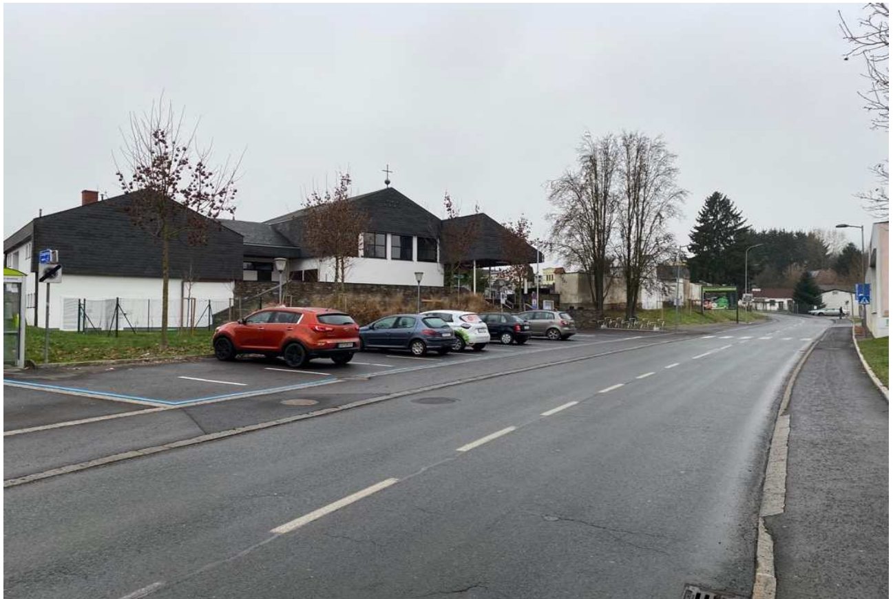
Fig. 4: Implementation site Oedter Straße, long-established street on the outskirts of the city
