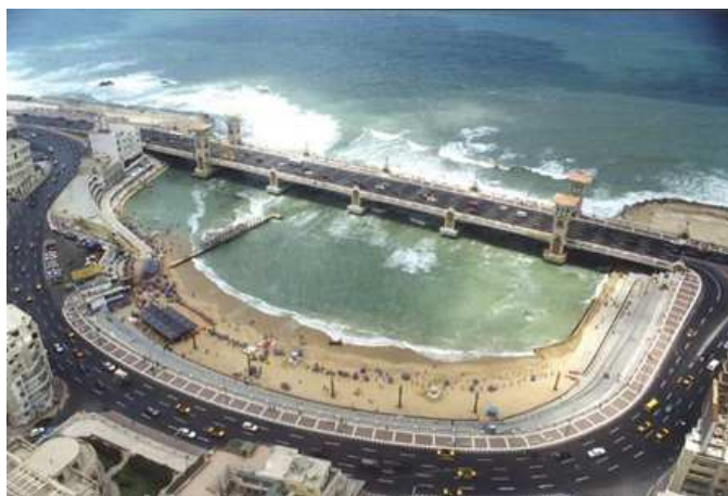
Fig. 5: View of Stanley Bridge, Alexandria, Egypt (Source: (The Arab Contractors, 2019)).
