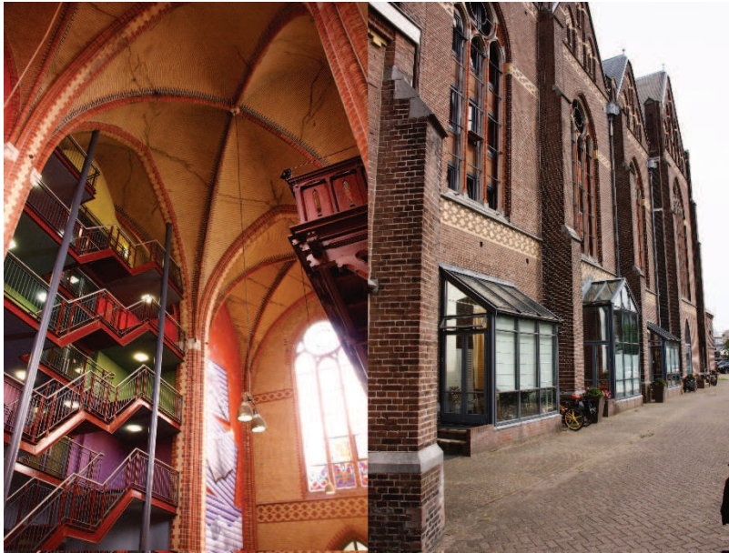
Fig.4: Two main consequences of a residential re-use can be found at examples like the Elbakerk in Haarlem (32). The addition of extra floors to create more ground space and also the addition of windows to ensure a sufficient lightning inside.
