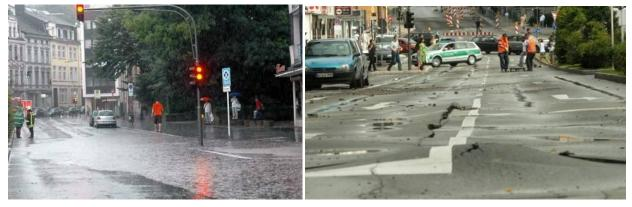
Figure 4: Damage due to uncontrolled storm water run-off.
