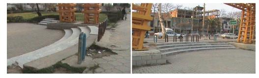
Figures 5 and 6: Park has stairs and bollards. There isn't any ramp for the disabled.
