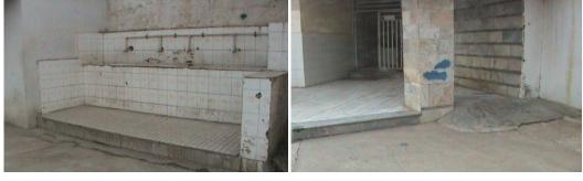
Figure 1: The public drinking-fountain is located on platform. Figure 2: The ramp in the public toilet isn't standard.
