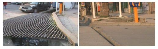
Figures 9 and 10: The junction point between pedestrian and street should be flat but in these pictures we are faced to some levels.
