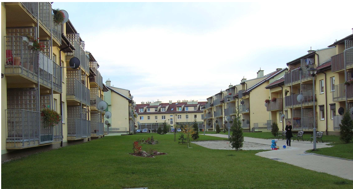
Fig. 1. Housing complex in Wrocław, Miłostowska St.
