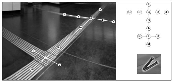
Fig. 3: The RFID-tags structure including the nesecarry links between these tags
