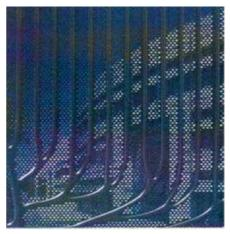
Fig.13: Transparent solar thermal facade collectors
